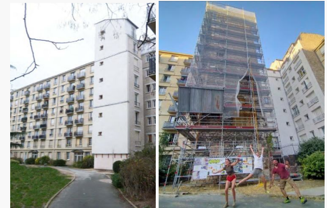
Pictures of the existing gable before and after work.
