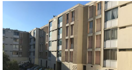
B – LARGE HOUSING ESTATES IN SUBURBAN AREAS
