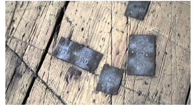
Mould loft – Nantes – The reused wooden floor bears imprints of the ship layout carried out in the old Dugigeon hall. Metal plates show the name of the ships.
