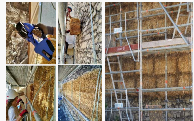
Focus on the implementation of straw bales on the building site
