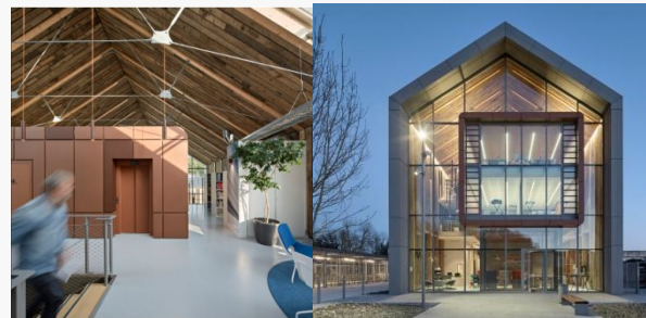
4 MOULD LOFT – IN SITU REUSE - AIA ENVIRONNEMENT, NANTES. The project includes reuse and highlighting of timber slats from the N+1 floor to cover the nave of the new bow on the town side with interior cladding. Beyond the generated saving of resources, this strategy shows a definite architectural and heritage interest: the floor still bears nominative ship metal plates which were designed in the former mould loft.
