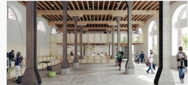
5 REHABILITATION OF THE MANUFACTURE DES TABACS AND EXTENSION OF THE G2E1 POLE – IN SITU REUSE - STRASBOURG – In this renovation project, the reuse of existing structural elements required strategy of reinforcement and differential treatment to insure their sustainability. Original façade joinery, framework, wooden floors and cast iron posts were thus refurbished and reused in situ.
