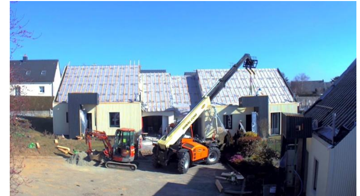
The "energiesprong" external insulation system for individual housing represents an opportunity to reduce emissions related to heating energy.
