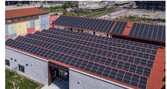
Solar sources strongly conditioned by urban morphology. The industrial heritage wasteland represents a substantial source without affecting the identity of the built asset.
