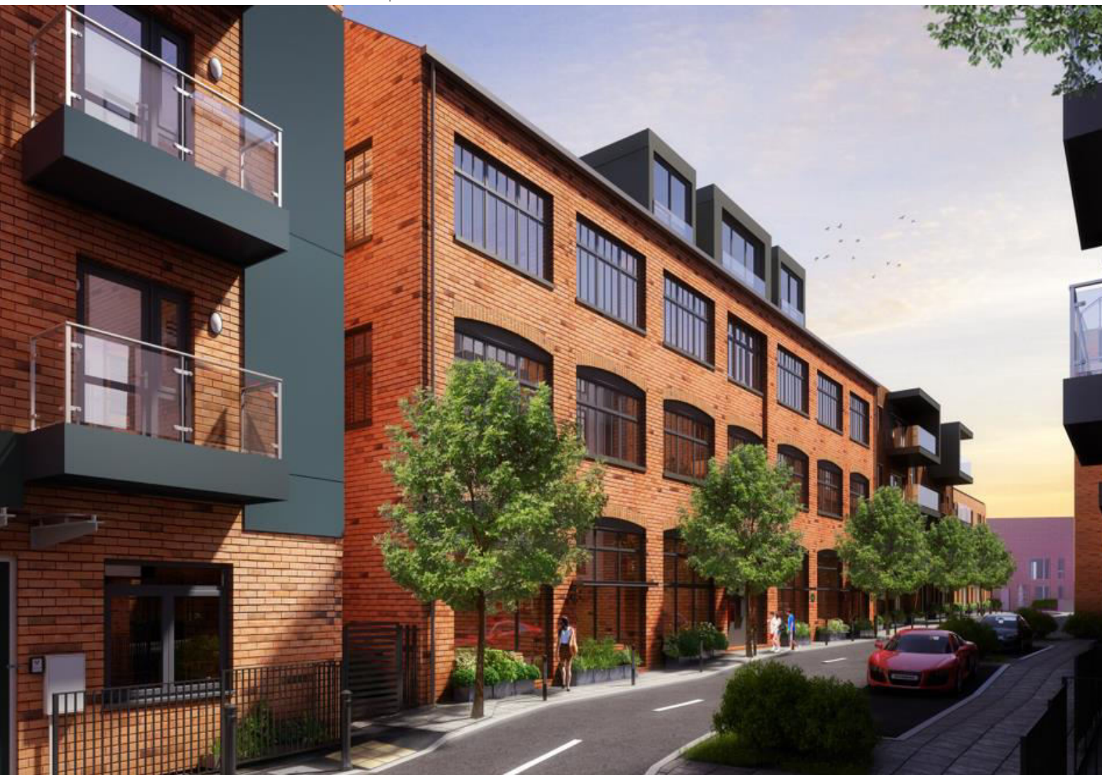
Figure 4 - Courtauld Road, London, mixed tenure housing scheme, refurbished Victorian warehouse. BREEAM Score 'Excellent' (80.69 per cent) and winner of the 2016 BREEAM Residential Award. (Source: BRE Global)
